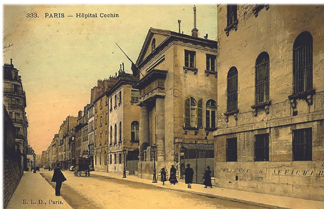
Fig. 7b, c : Foch Hospital and Cochin Hospital.
